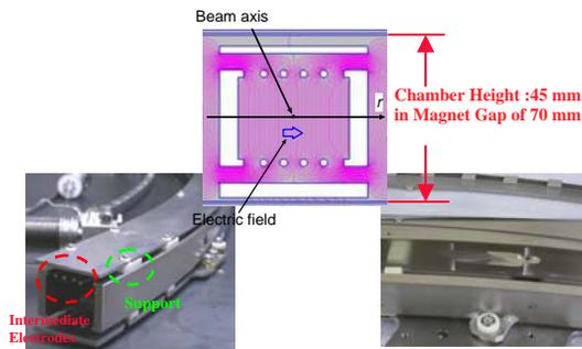
Fig. 6 Electrodes installed into each dipole magnet of S-LSR to suppress “shear heating.”
